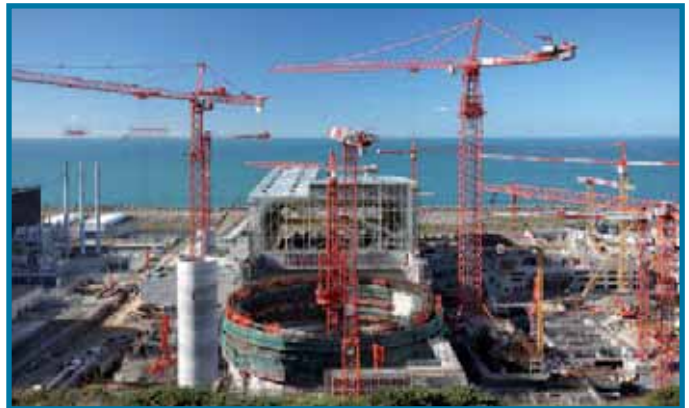
Fig. 3. General view of Flammanville 3 being constructed October 2009.
