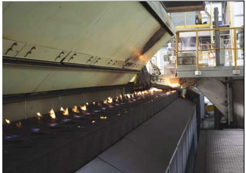
With an output of 330 moulds per hour and a high yield percentage, the DISA 240-C is a successful addition to the Pohang foundry plant
